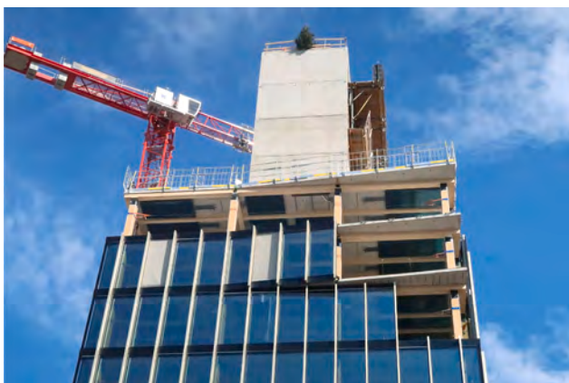
Fig. 2. View of the building Arbo during construction with already completed concrete core and subsequent timber construction.
